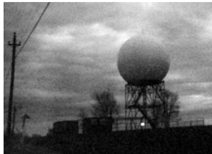
Radar guidance system at Fort Campbell – sitting on a grounding system of a gas line, power line, railroad tracks and smaller electrical distribution line.
