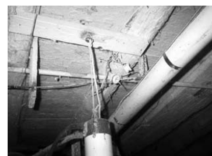
Trainer isolator located in a mess of wires, metals, pipelines and automatic take-off. All covered with whitewash which gets moist in summer
