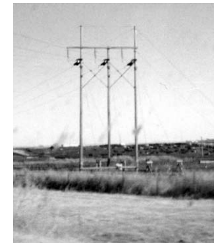
Transpositioning over concrete interstate highway.
