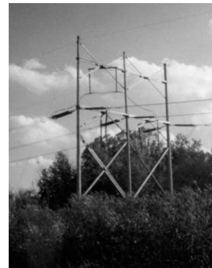
Transpositioning over gas line and a very marshy area.
