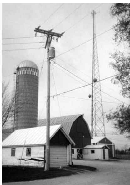
Cell tower behind farm capacitor (by drive) with barn in-between
