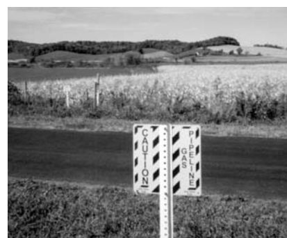
Yellow sign denoting buried gas pipeline
