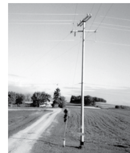
Close-up of steel pole
