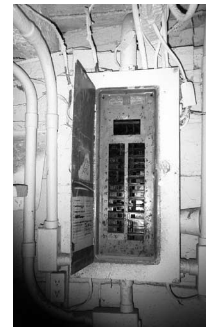
Newer, updated set up, 200 amp service in conduit. Barn is split. Box on left serves silos, gutter cleaner and fans. Box on right with fire extinguisher services the milk house and all equipment in that area – doors always closed.
