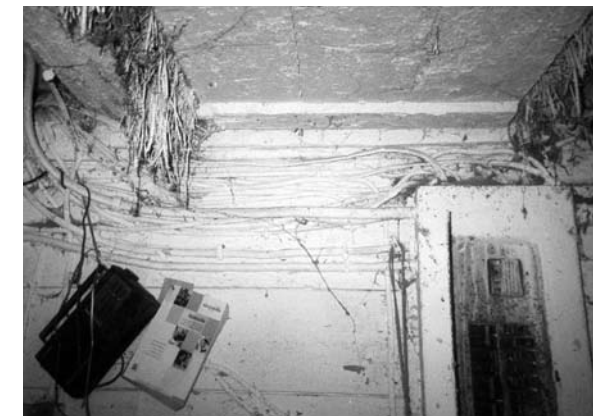
Old entrance box, miles of Romex, spider infested, damp box.
