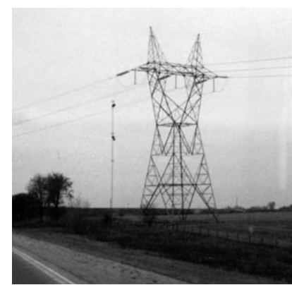
Transpositioning next to a cell tower.
