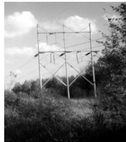
Transpositioning flipping the charge over a gas line.
