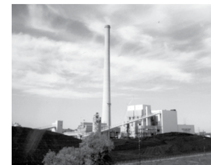
Electrical generating plant
