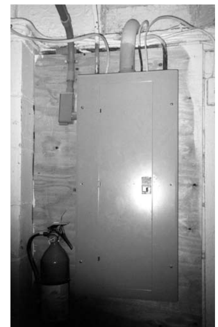
Newer, updated set up, 200 amp service in conduit. Barn is split. Box on left serves silos, gutter cleaner and fans. Box on right with fire extinguisher services the milk house and all equipment in that area – doors always closed.
