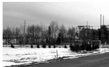
A second picture of the same farm that shows a little more about why they have problems with stray currents. As this photo shows plainly, there is a power substation just a few hundred feet NW of the barn. Also, a manure lagoon sits between the barn and the substation making matters worse (Manure pits contain a lot of ions potassium, sodium, chloride, etc. that cause them to act like a large battery).
