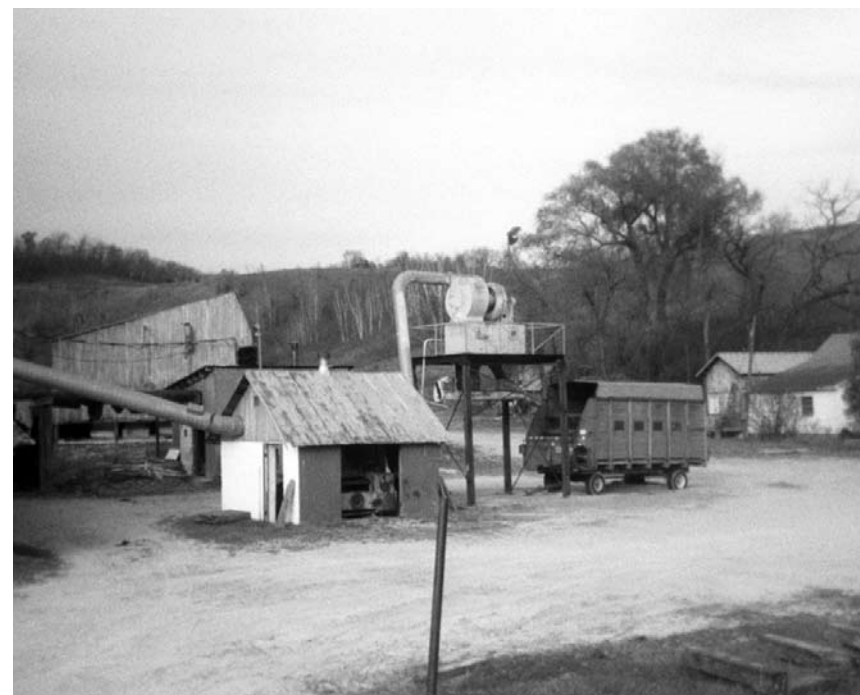
Diesel generator – keep ground away from barn.
