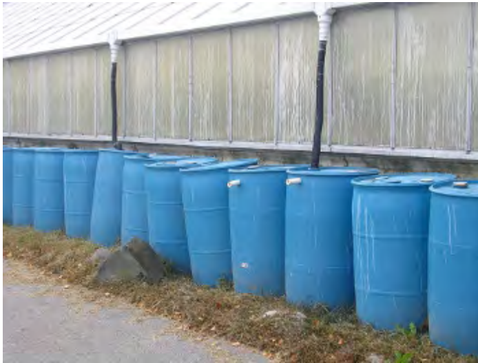
The Mt. Auburn Cemetery in Watertown, MA collects the majority of its water for irrigation from rain barrels off of the roof of its greenhouse. Each barrel is connected to the next via plastic tubing. This means when one rain barrel is full, it overflows into the next barrel, and then the next. It's a clever system for capturing a large amount of rainwater for later use. Photo from Paul Kwiatkowski at Mount Auburn Cemetery.
